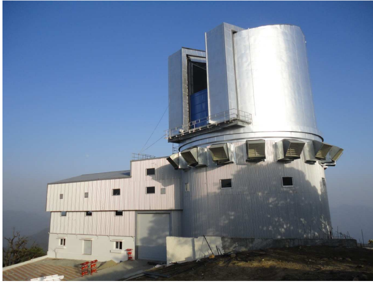
Figure 1. The enclosure of 3.6m DOT facility at Devasthal. The wind screen is seen in blue color.
